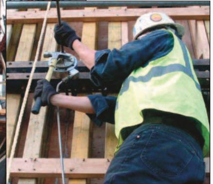
At the heart of many construction projects is a rebar-reinforced concrete structure holding it up. Support columns and walls begin as rebar 'skeletons' around which the concrete is poured. Wood or fiberglass forms are built around the rebar framework and concrete is poured into the cavity. The forms hold the concrete in place until it hardens, then are removed.
