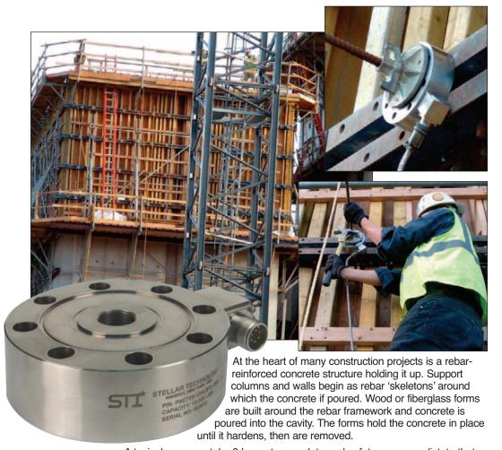
A typical pour can take 8 hours to complete and safety concerns dictate that the concrete be introduced slowly to give it time to set up and become self supporting before more is added. Adding too much concrete too quickly could result in the forms failing under the weight.
